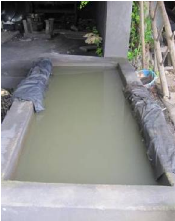
Pic 16. Wastewater will discharge directly to
